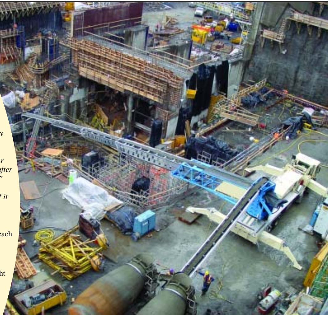
Kiewit uses the TB 130 on a powerhouse pour in Grand-Mere, Quebec on December 6, 2001. The unit placed 425 cubic yards of 2.5" aggregate at a 2" to 3" slump concrete.
