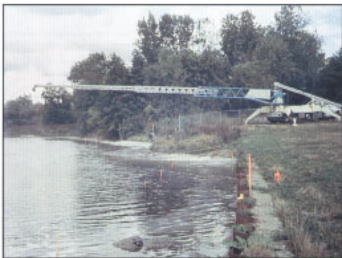
TB 105 operating from the shores of the Ottawa River.
