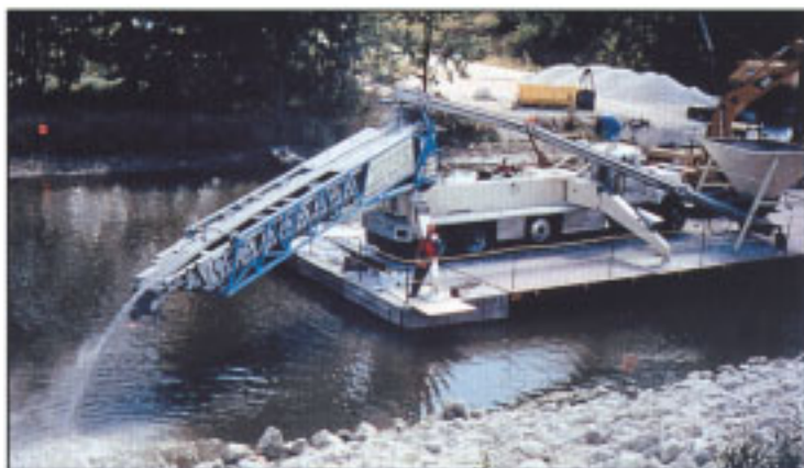
An excavator keeps the hopper of the TB 105 filled with AquaBlok.
