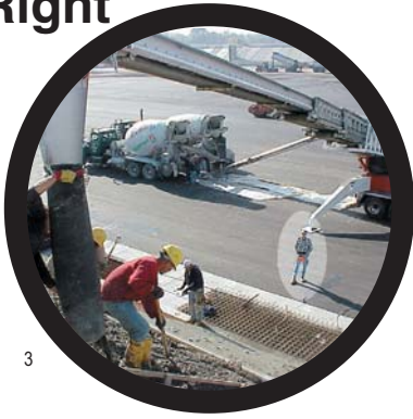
Above: Correct approach with the operator at a strategic “V” position between hopper and main boom.
