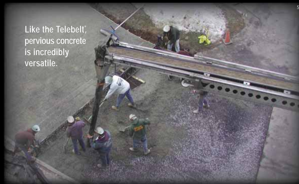
Engelman Construction turned to a Putzmeister Telebelt® TB 110 for help to place 40 yards of pervious concrete on this Fogelsville, PA, job site. The parking lot pour, one of many applications pervious concrete is used for, took a total of three hours to complete.
