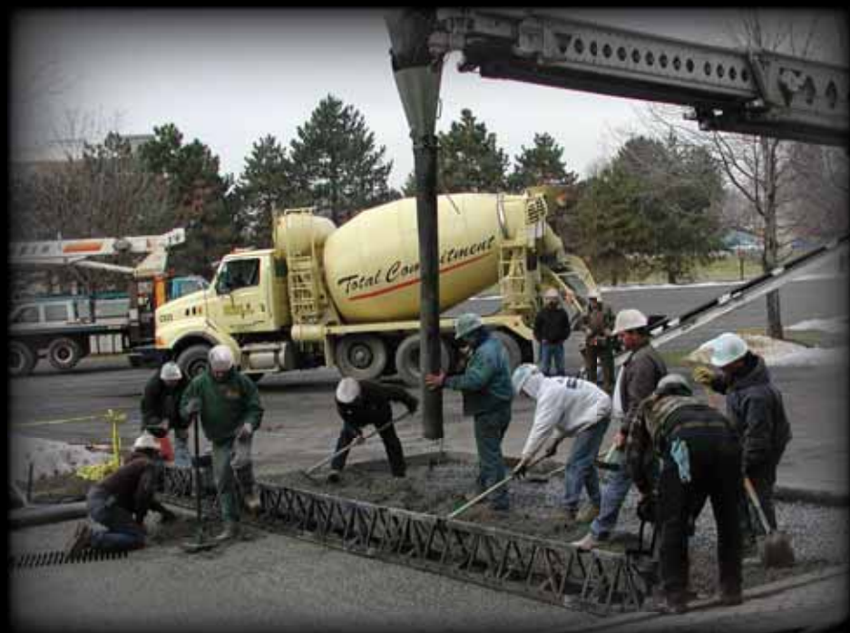
The Engelman team only had to position the Telebelt® TB 110 at one location for the entire pour with no remobilization necessary.
