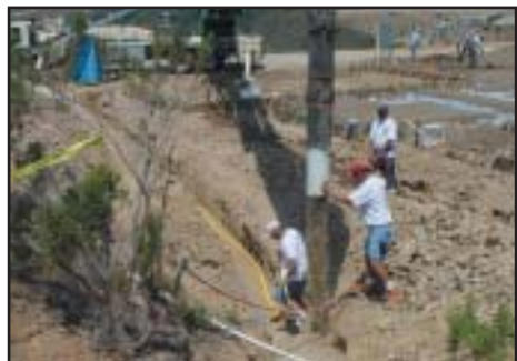
Utility trench backfill
