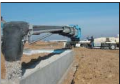
Drainage stone - foundation
