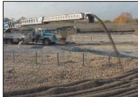
Aggregate on settling basin
